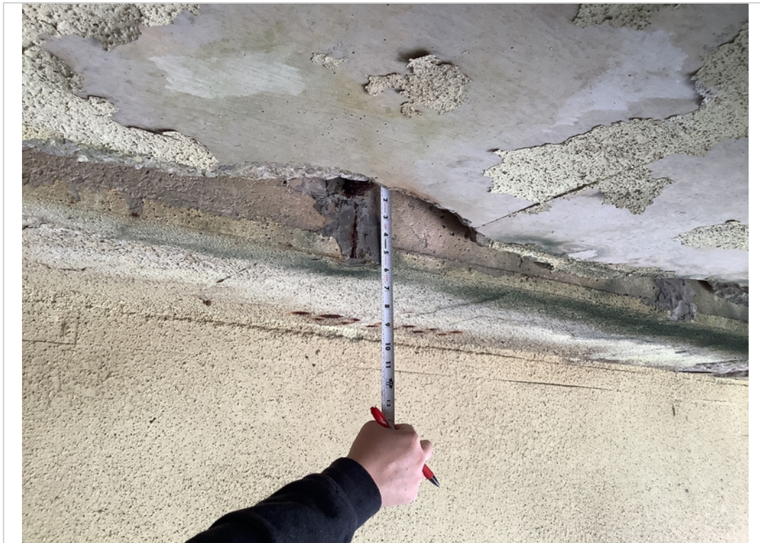
Typical moderate spall in bottom of deck
