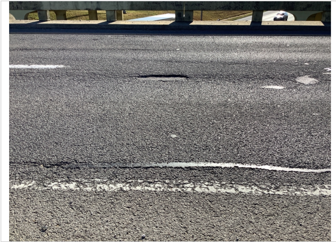
Typical pothole in wearing surface
