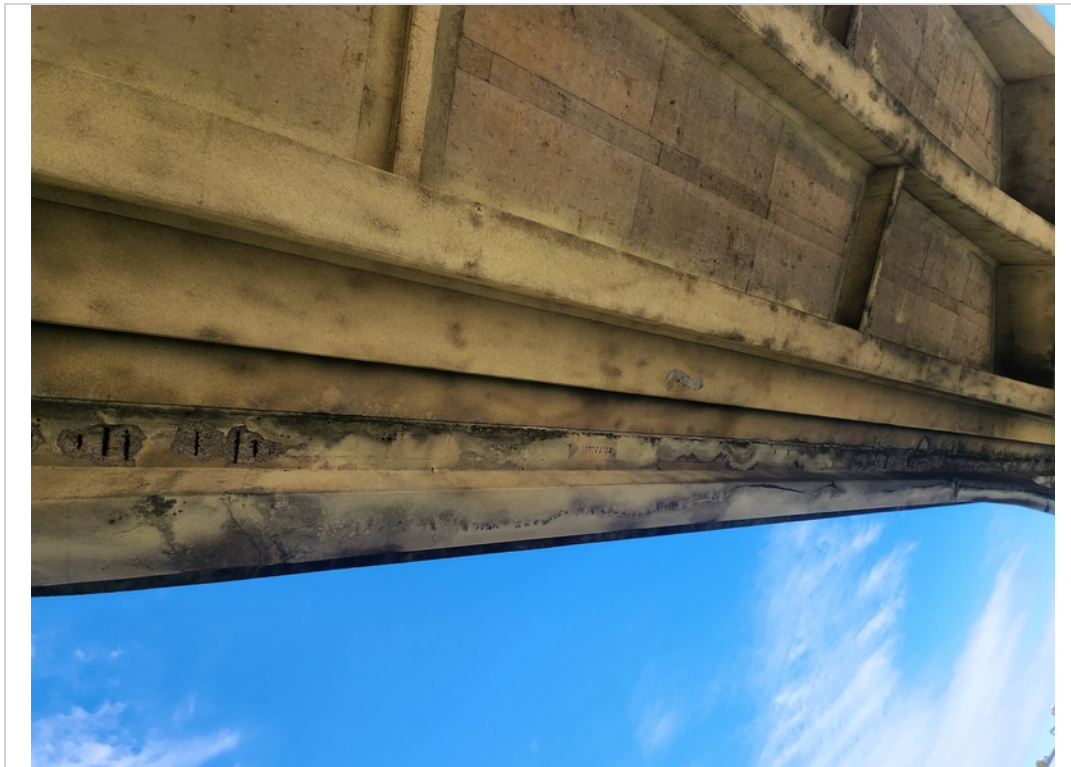
Hairline longitudinal crack along length of beam "A" in span #3
