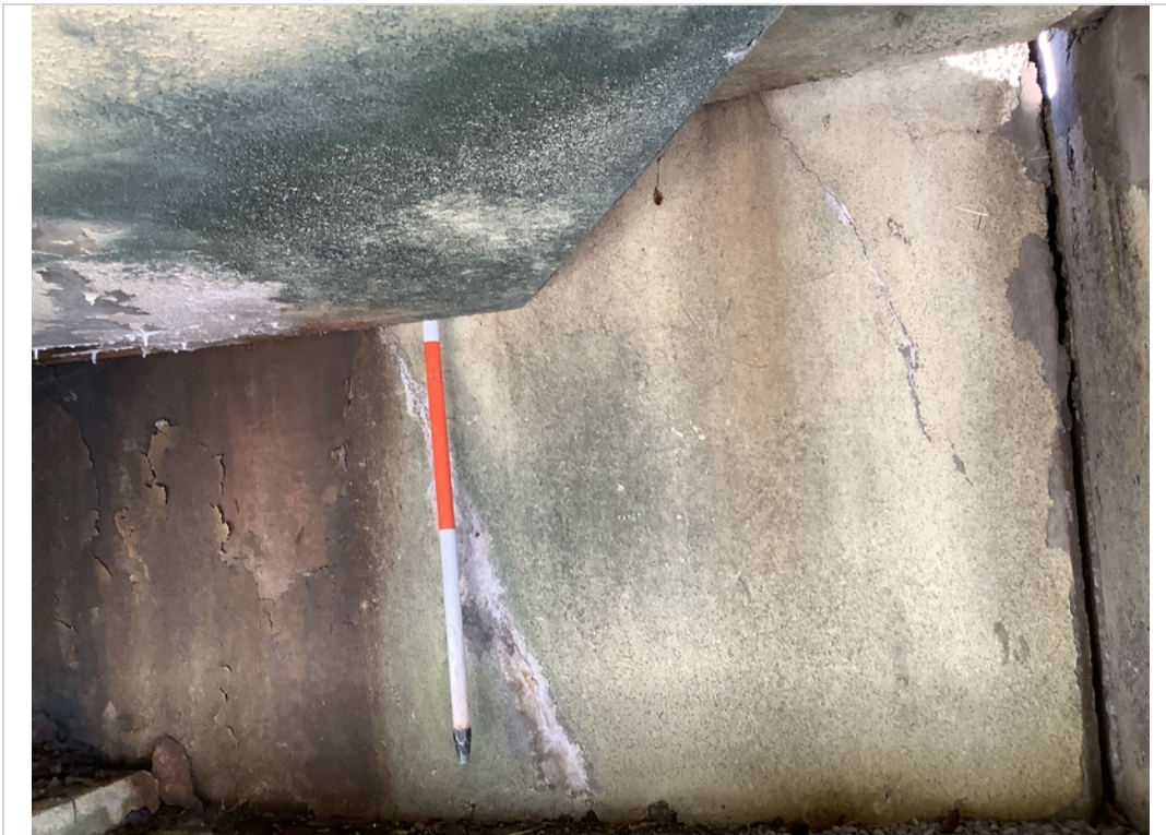
Void between deck and abutment #1 at left side
