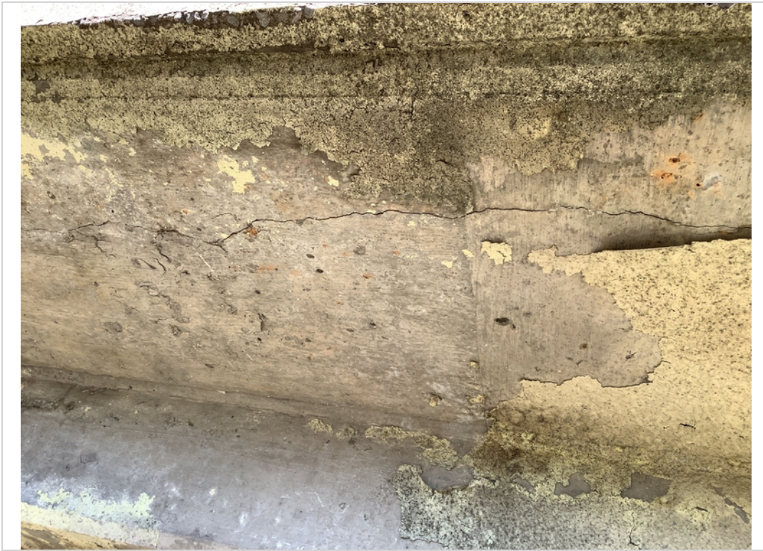
Typical crack in bottom of deck
