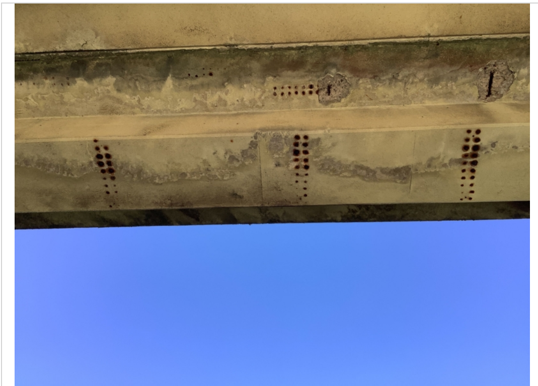
Typical rust staining in bottom of deck
