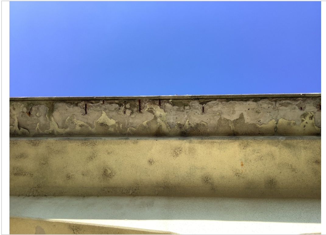
Typical spalls with rebar in right overhangs
