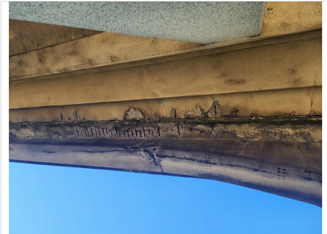
Typical moderate spalls with exposed rebar in bottom of deck bay "A"
