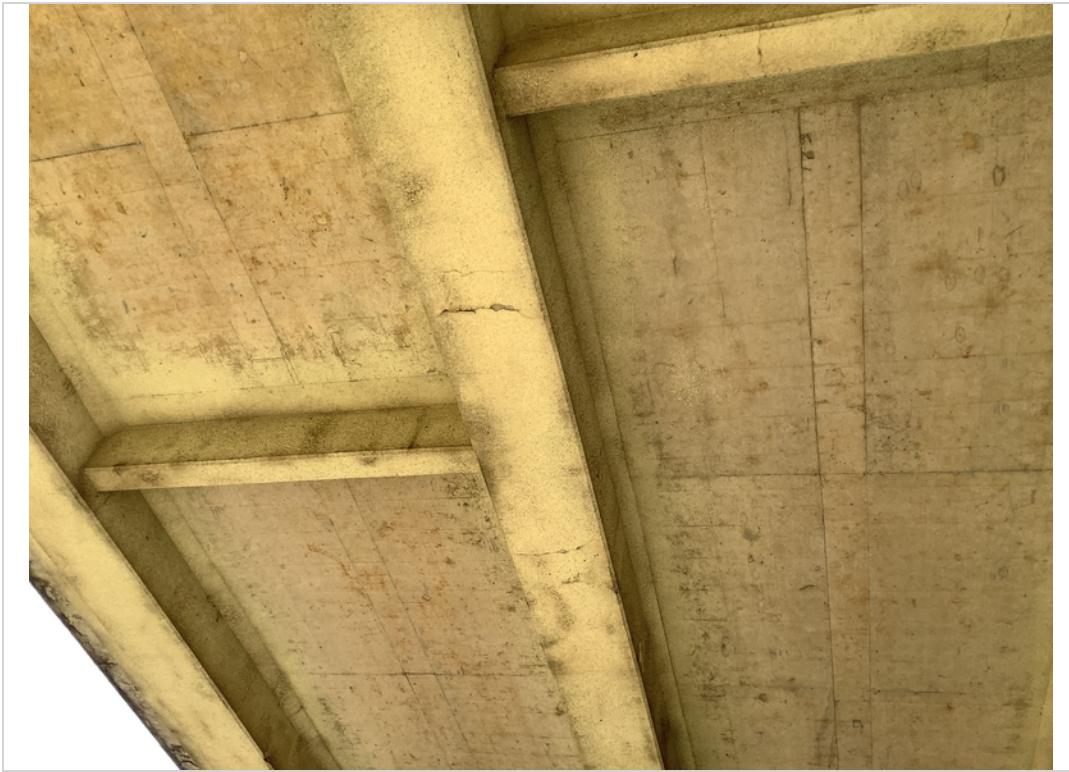
Typical cracks on beams
