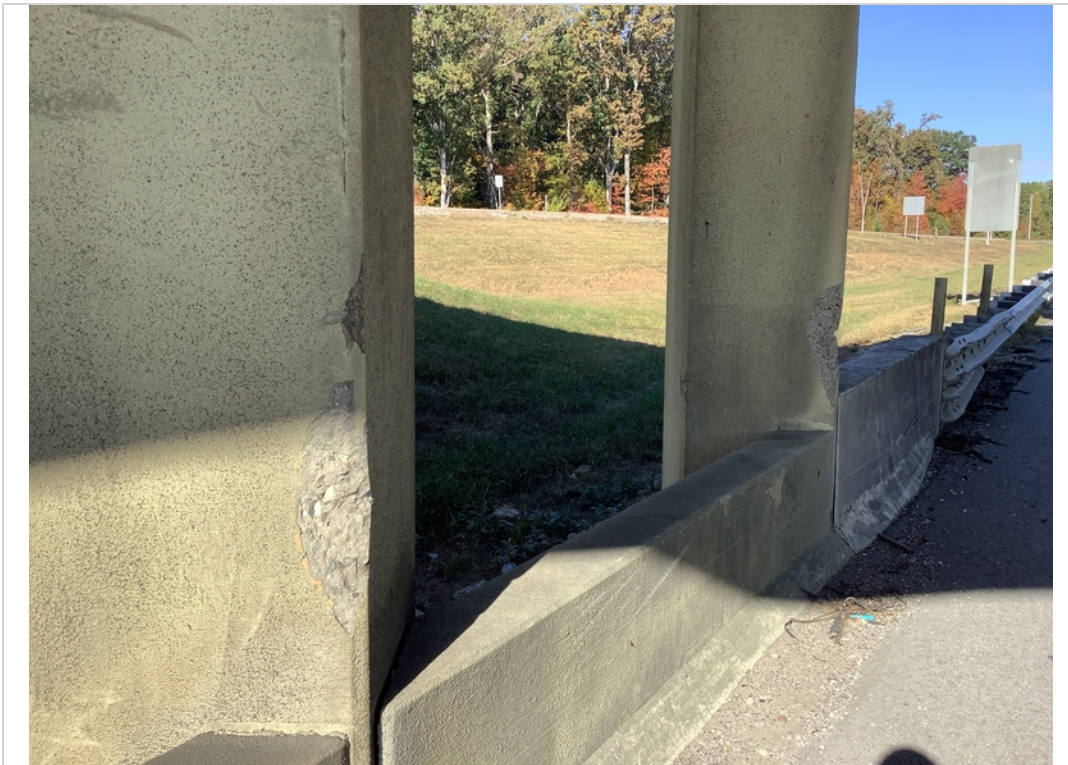
Typical spalls on bent columns from collision damage
