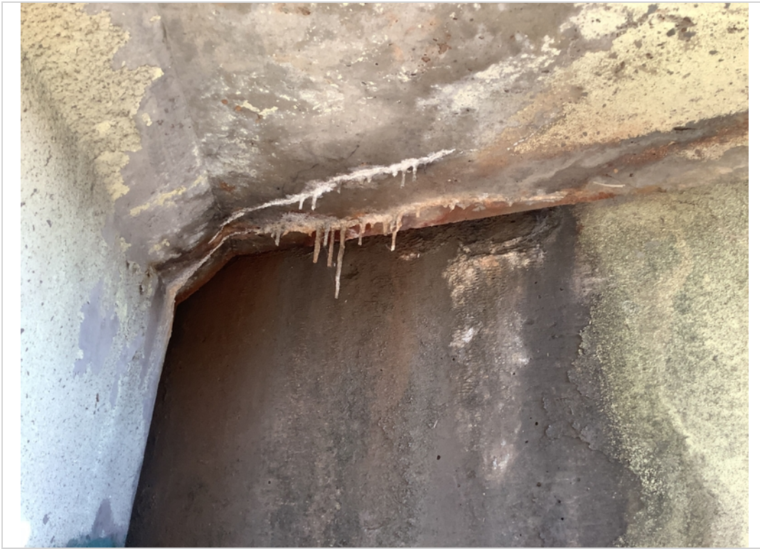
Typical moderate efflorescence in bottom of deck
