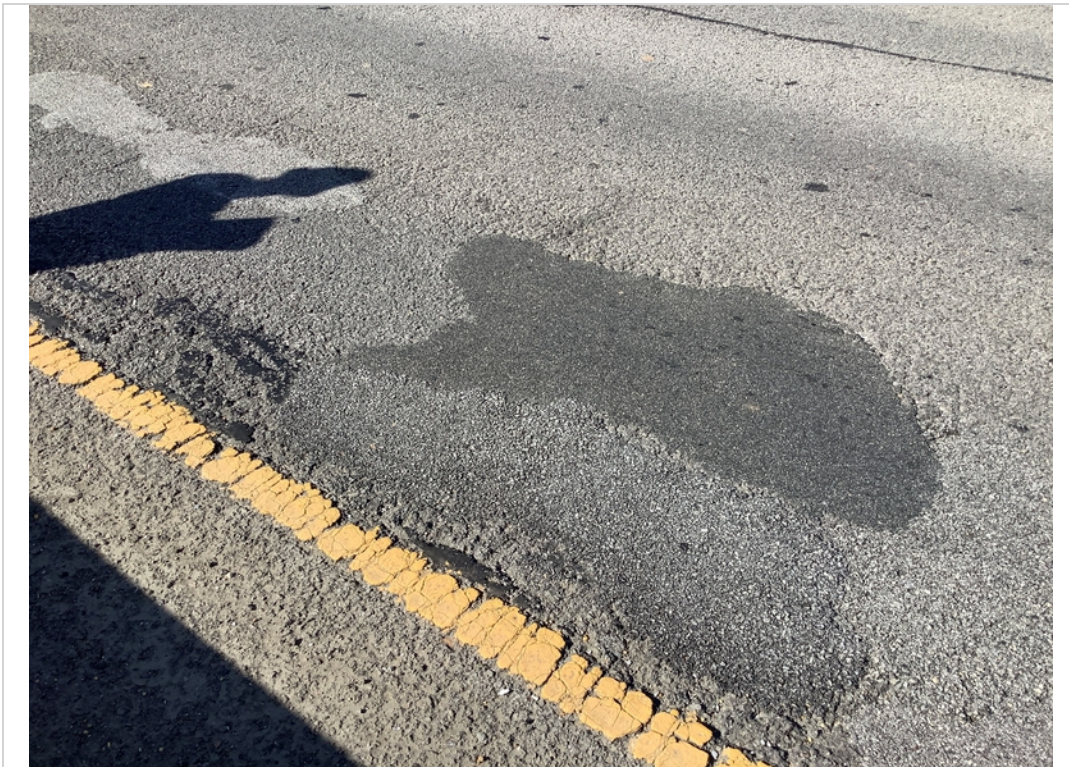
Typical rough and uneven wearing surface
