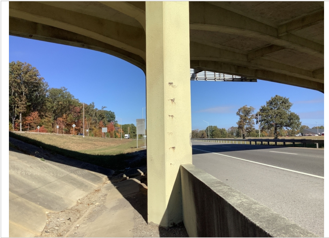
Typical rebar pop-outs on bent columns
