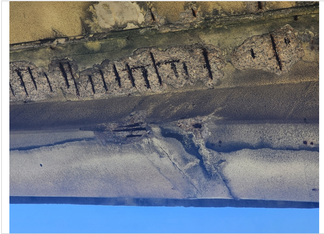
Moderate spall on beam "A" in span #3 with exposed strands
