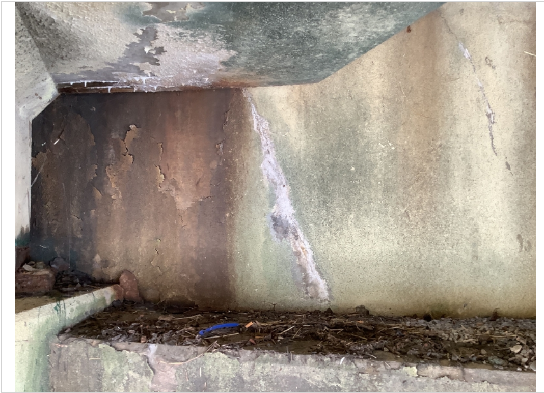
Typical cracks with efflorescence at abutments
