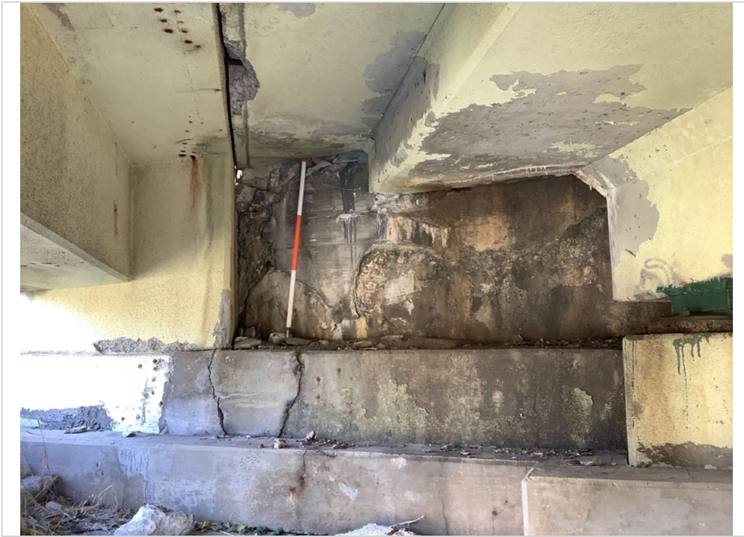
Void between deck and abutment #2 at left side
