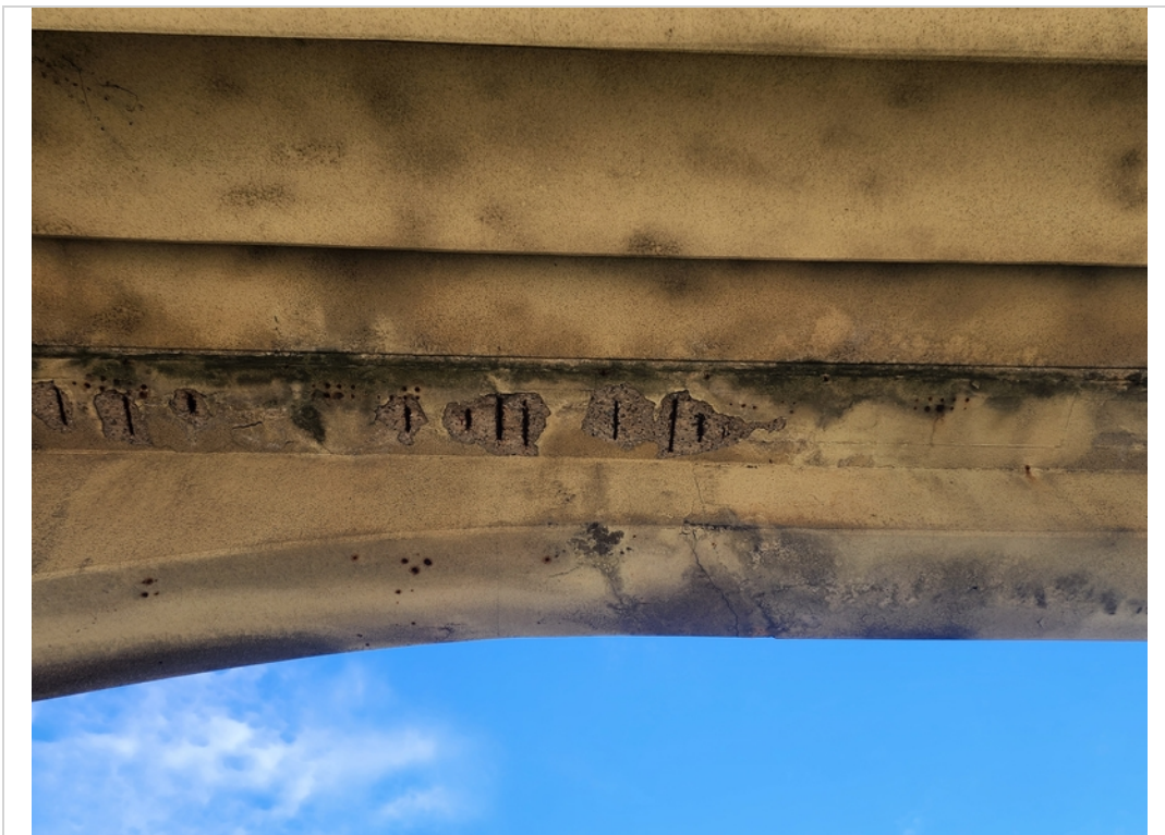
Moderate vertical crack in beam "A" in span #3
